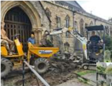
Making the level platform
