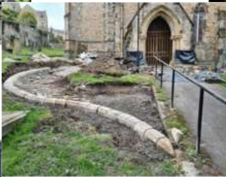
Creation of curved ramp
