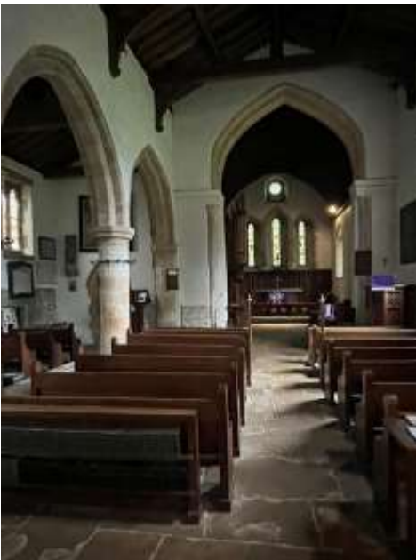
Nave of the Minster
